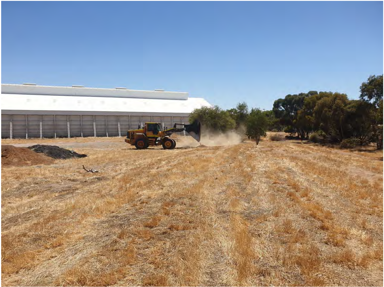
Photograph 1: General view of proposed accommodation site looking north
