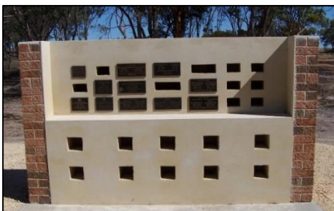
Harrismith Niche Wall
