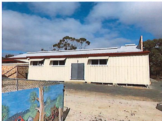
Harrismith Hall exterior has been painted as part of the 2019/20 budget
