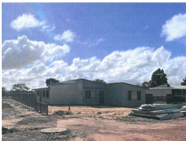
Progress of new Executive Residence at 14 Smith St, Wickepin.
