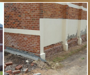
Old Road Board Building Restoration
